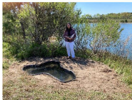
Paula is happy with the installation of the form.
