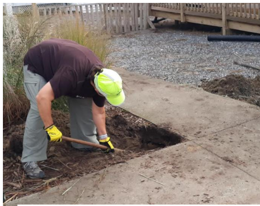
Excavating under the sidewalk for the outflow
